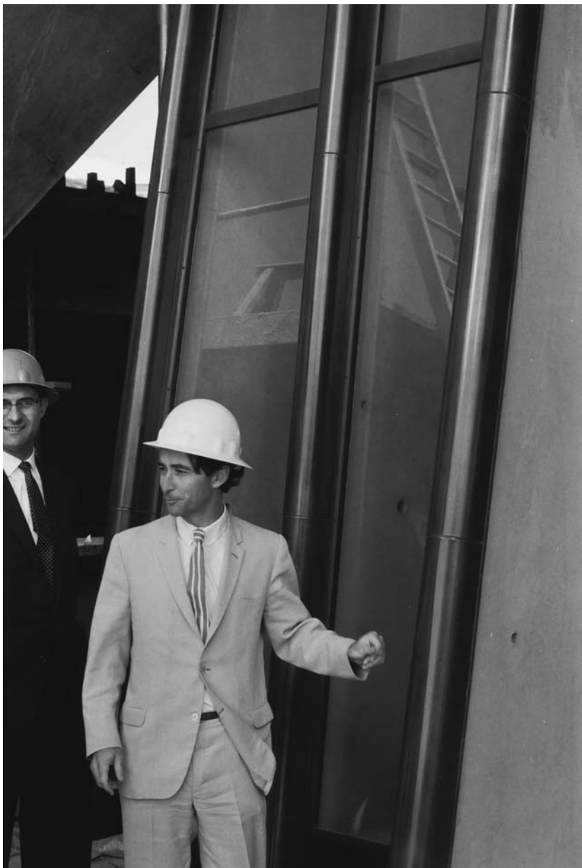
Figure 3: Peter Hall and an on-site glass wall prototype showing the first bronze-capped, concrete mullion scheme, abandoned in late 1967. Peter Hall Papers.
